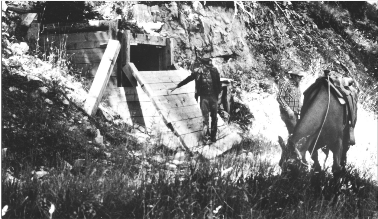
Figure 154. Abandoned Taylor Creek Adit, date and individuals unknown. BLM file photo.
